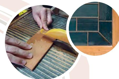
We recommend using a wet saw with the glazed side down. If any chips occur it will be on the back not the glazed side.
