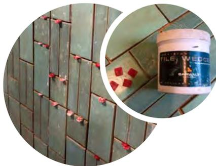
For spacing out tiles we recommend wedge spacers. They come in many different sizes to accommodate both historic and handmade tile. They also help prevent tile slippage on vertical surfaces.
