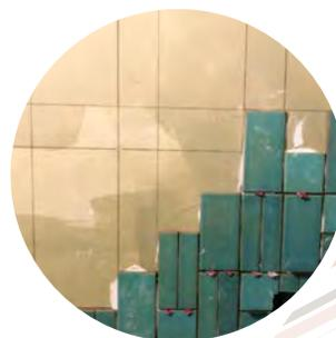
Lay out the tiles for your project. Make sure they fit your measurements, and arrange them to enhance the variation. Making guildleing on the wall using a laser guide or chalk line will help you keep the tiles straight and level.
