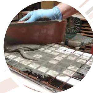
Wear rubber gloves. Force grout diagonally into joints with a rubber grout float. Ensure joints are completely filled. Wipe clean with a towel until grout haze is entirely gone. **Use very minimal or no water to clean grout.**
