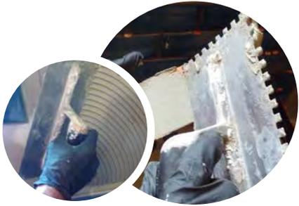
Use a notched trowel to spread mortar mixture across the prepared surface, creating combed rows. To guarantee full coverage “back butter” the tiles (thinly apply mortar to the tile back). When pressed into the combed rows it will suction to the wall or floor making it very secure from movement or sliding.
